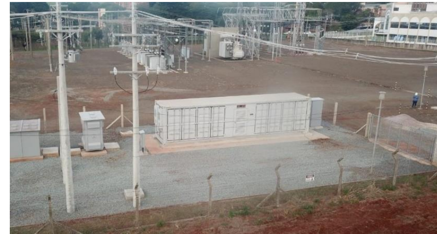
Barao Geraldo HV/MV Substation
