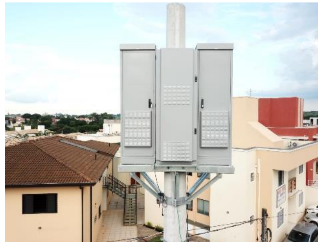
Pole mounted - applications in LV circuits
